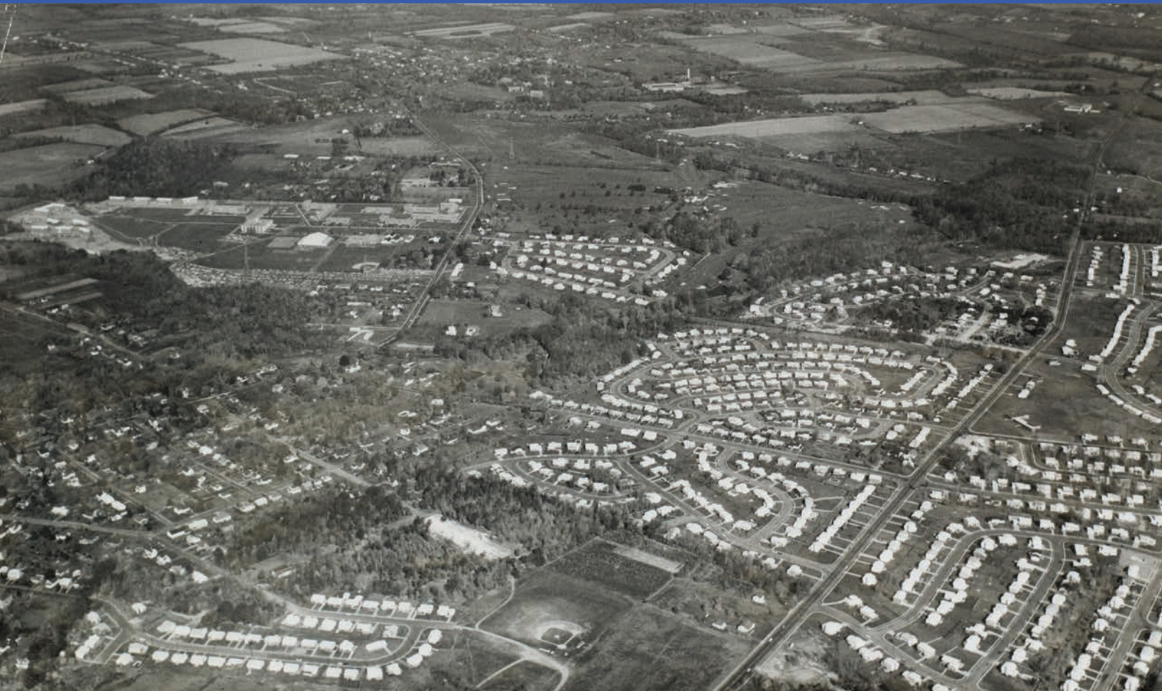
This 1963 photo of central Lawrence shows the new subdivisions of Nassau Estates, Norgate, Nassau II, University Park, and Pine Knoll.
