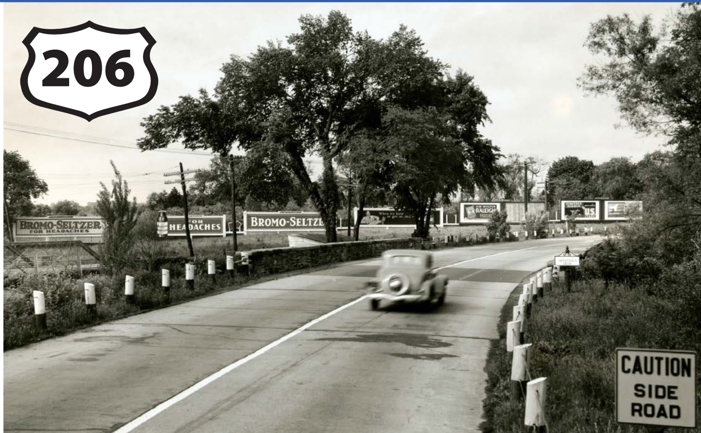
A driver crosses the new bridge over Shipetaukin Creek in 1934.
